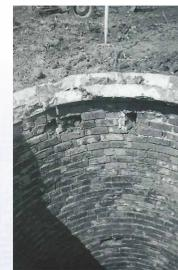
The mine was ventilated by a bricked air shaft which was about 12 feet in diameter and 120 feet deep. A fire would have been lit at the bottom of the shaft to create a draught in order to supply fresh air to the mine.
